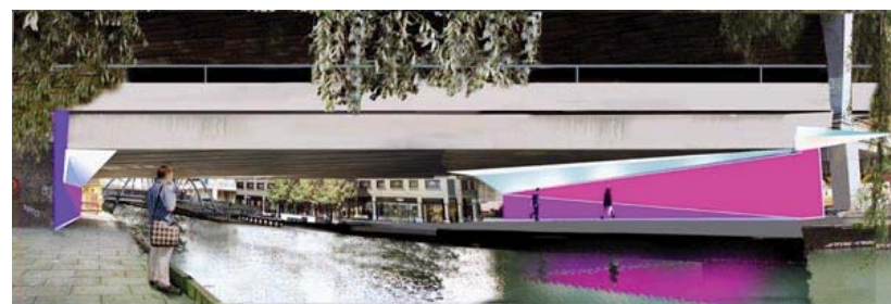
Infrastructure Lighting Installations
