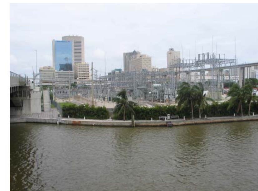
Existing: FPL Substation
